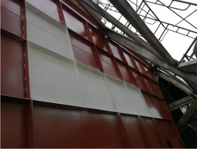
PSCoat can be applied directly onto the hot surface – without stop operation (till 150 C)
